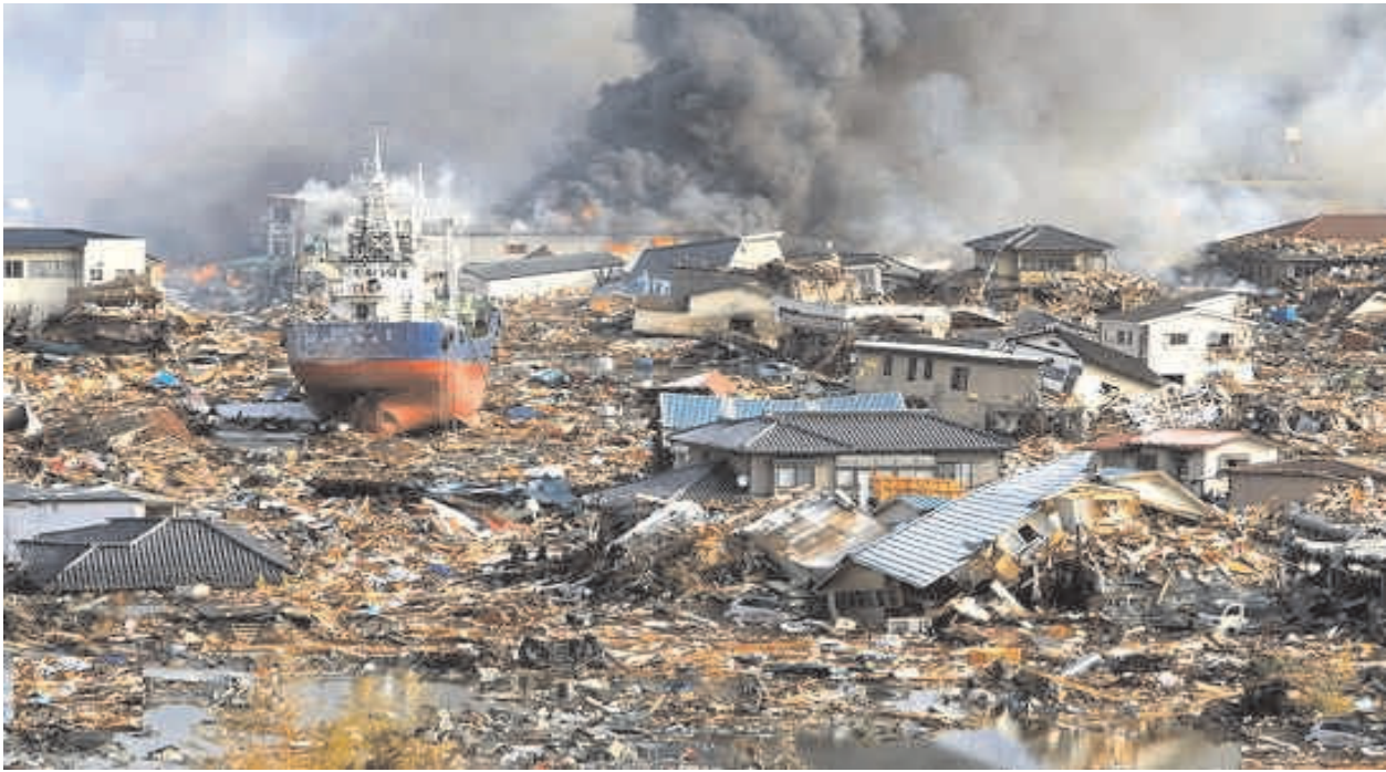
Figure 3: Mobile infrastructure destroyed in a disaster
